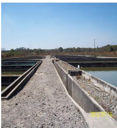
(i) Semi – concrete ponds
