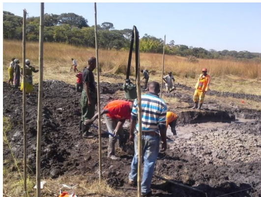
Pond pegging and Construction
