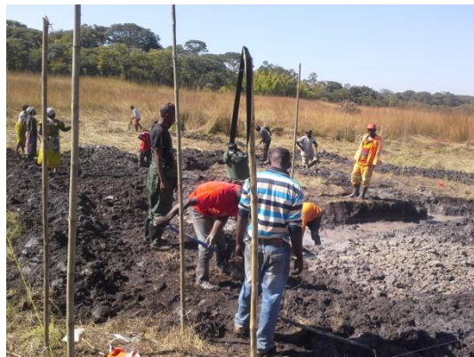
Pond pegging and Construction
